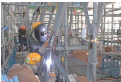
鉄骨溶接補修 (H29.11)
